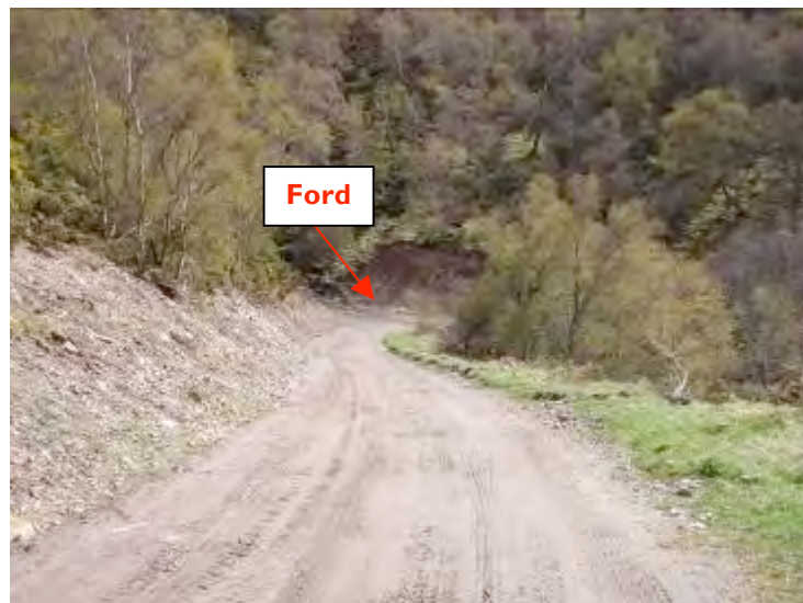
Fig. 4 : Works location 2 (photo taken April 2010)
